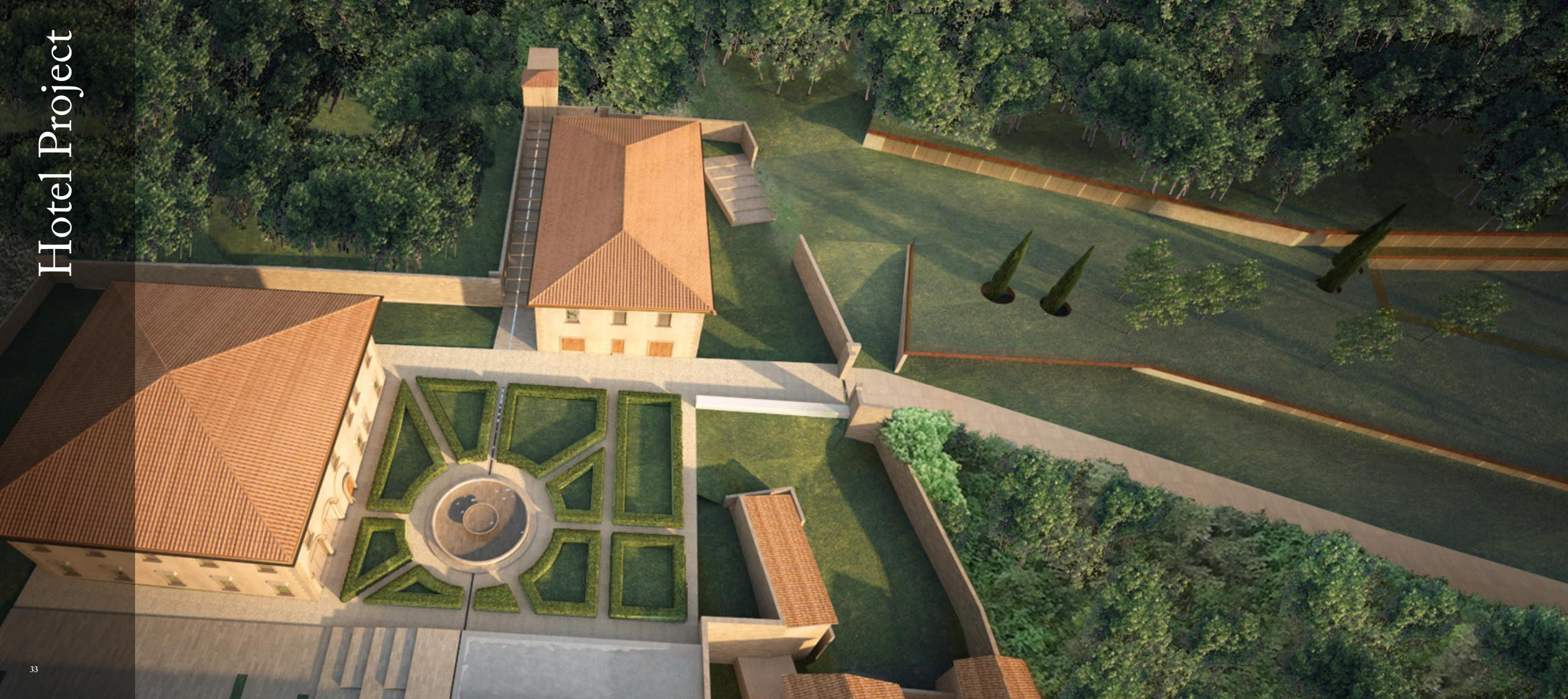
The Hotel Project is made by four blocks: Villa, Farm and Annexes which already exist, together with the new building, which includes an underground parking and two levels of rooms. These four units are linked at the underground level. The underground pathway is also equipped with small shops and with a conference room and it will be used every time, even if the surface road will be surely more pleasant and rewarding.
